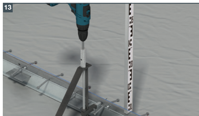
Check the height and adjust it using the screw on the jack.
